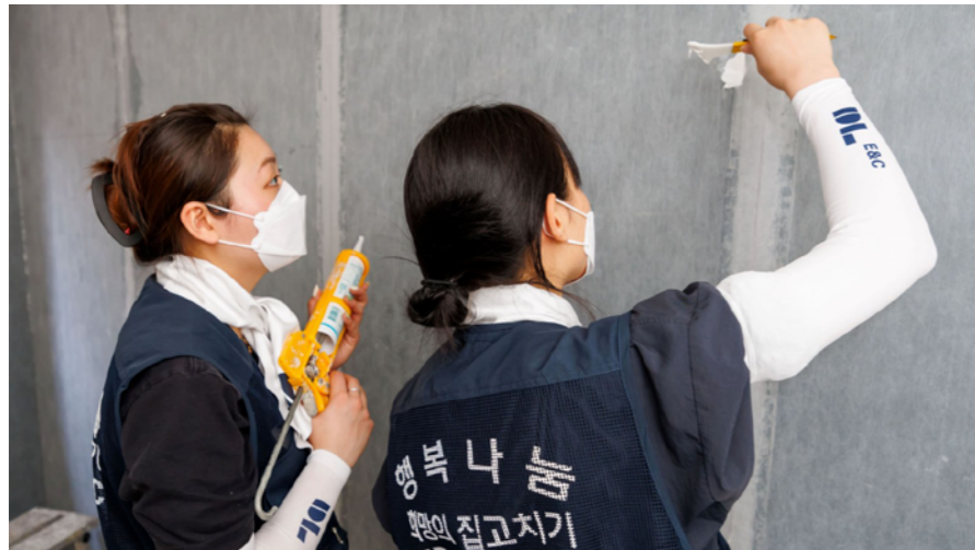
Repair house for hope
